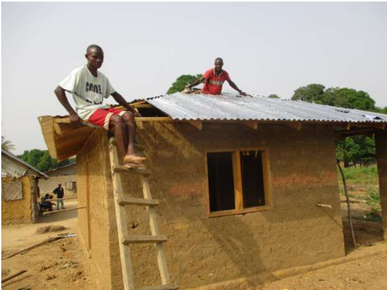
Member of Tappita Group KUU working on Food Storage Facility.
