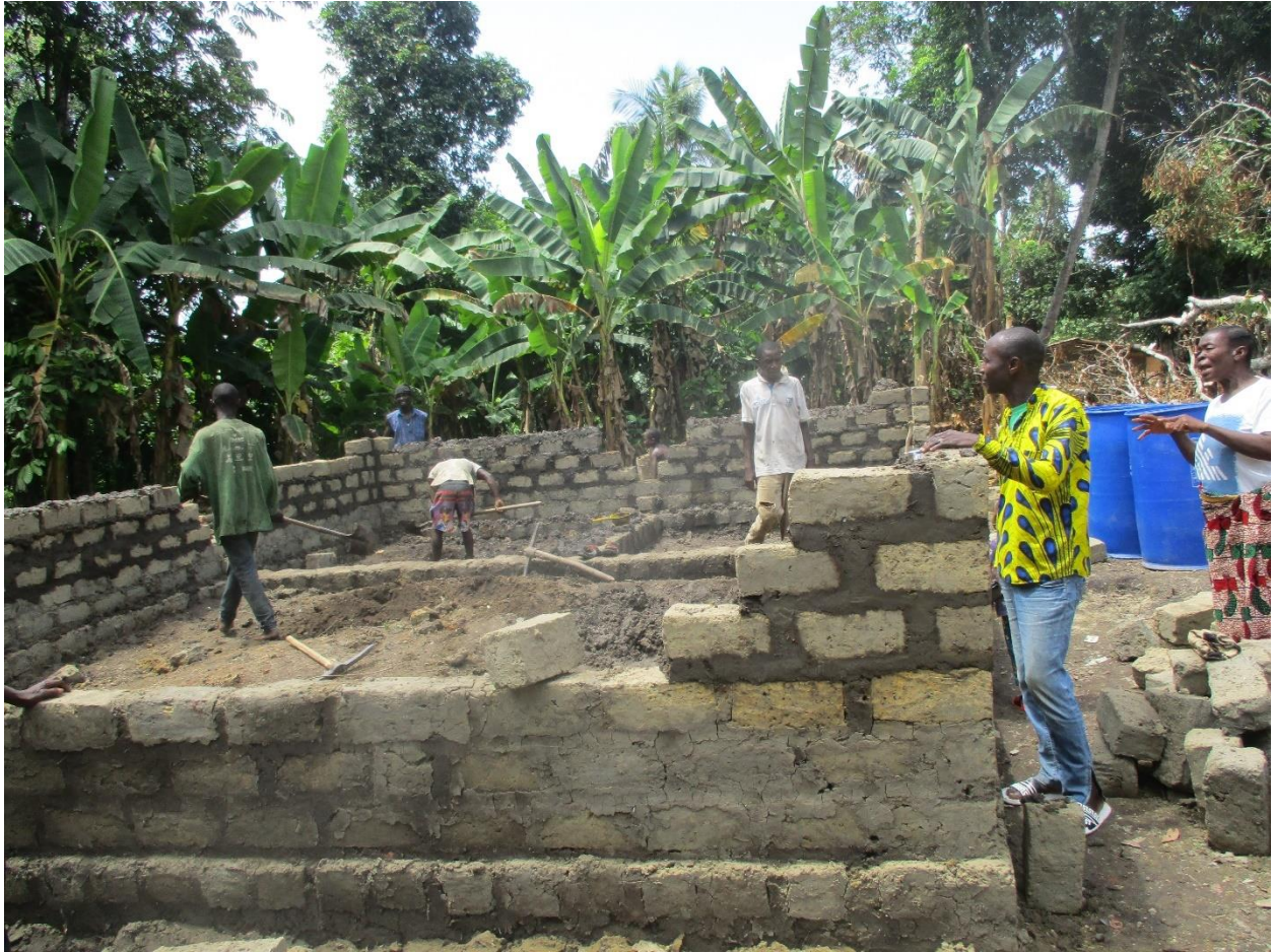
Liberia- Construction of Grain Store
