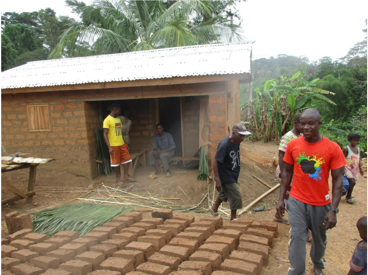
Liberia: Drying of bricks for construction of Grain Store
