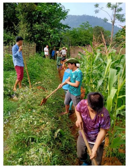
dig the pipeline trenches and transport building materials. Additionally, each family agreed to a \$13 fee to buy a water meter and smaller pipe to connect the main pipe to their house.
